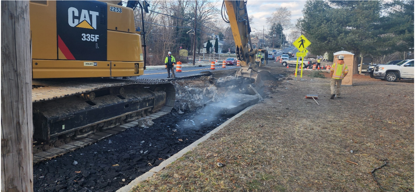
Figure 2: Removal of concrete pavement
