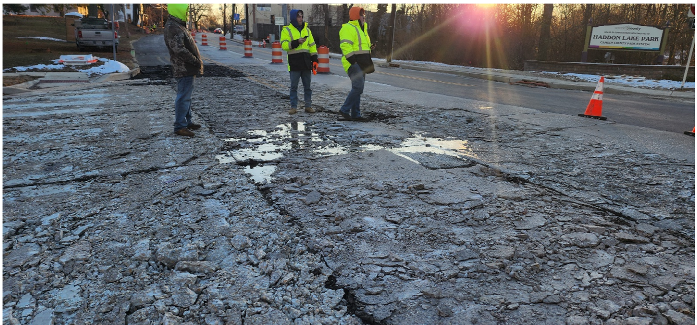
Figure:1 Rubblization of segment 3 westbound lane
