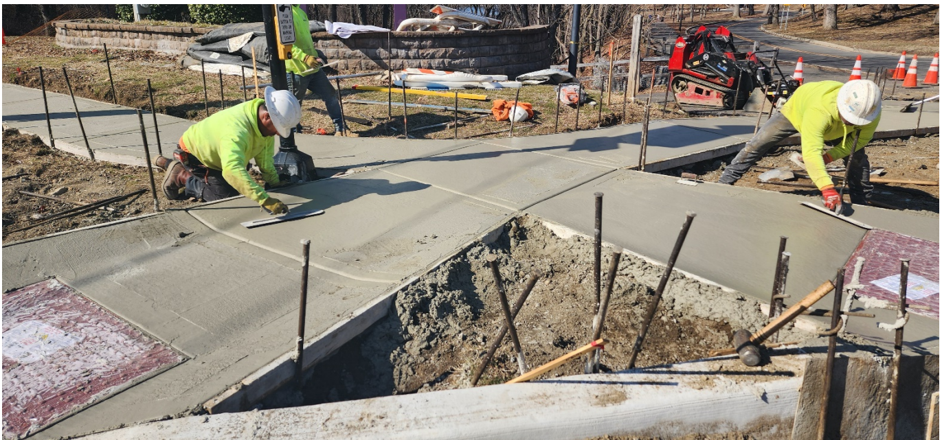
Figure 3: Concrete sidewalk installation in progress
