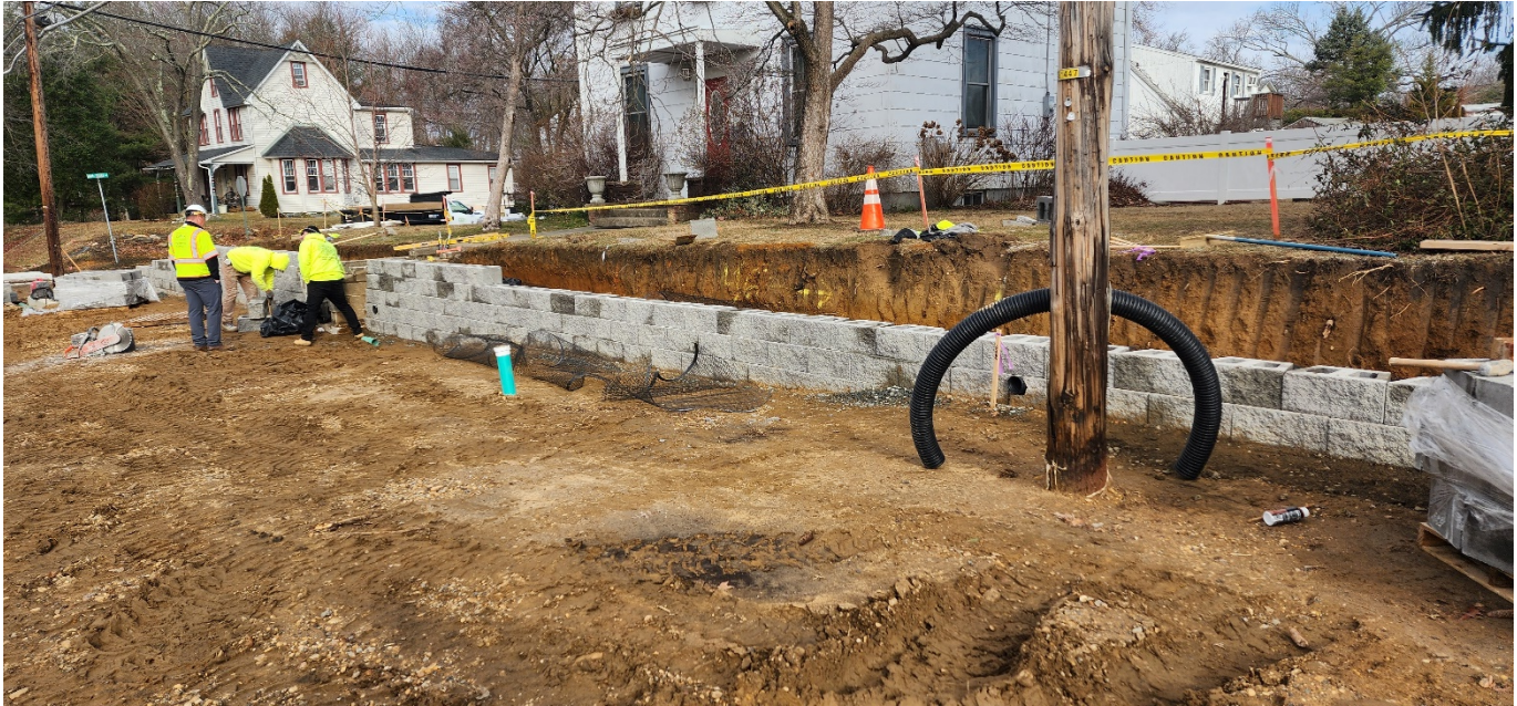
Figure 6: Retaining wall installation at the corner of Hampshire
