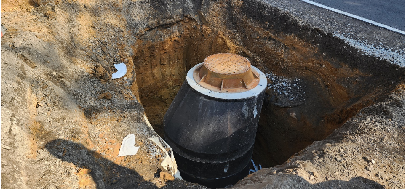
Figure 2: New sanitary manhole
