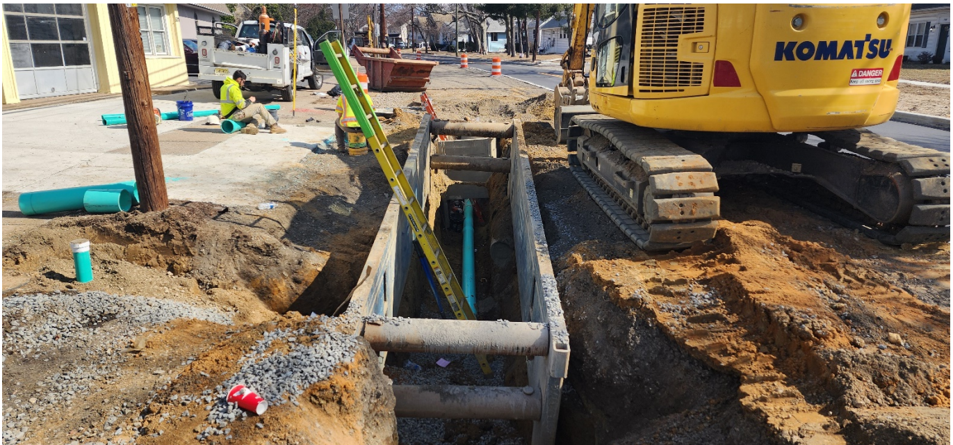
Figure 1: Sewer main Replacement in progress
