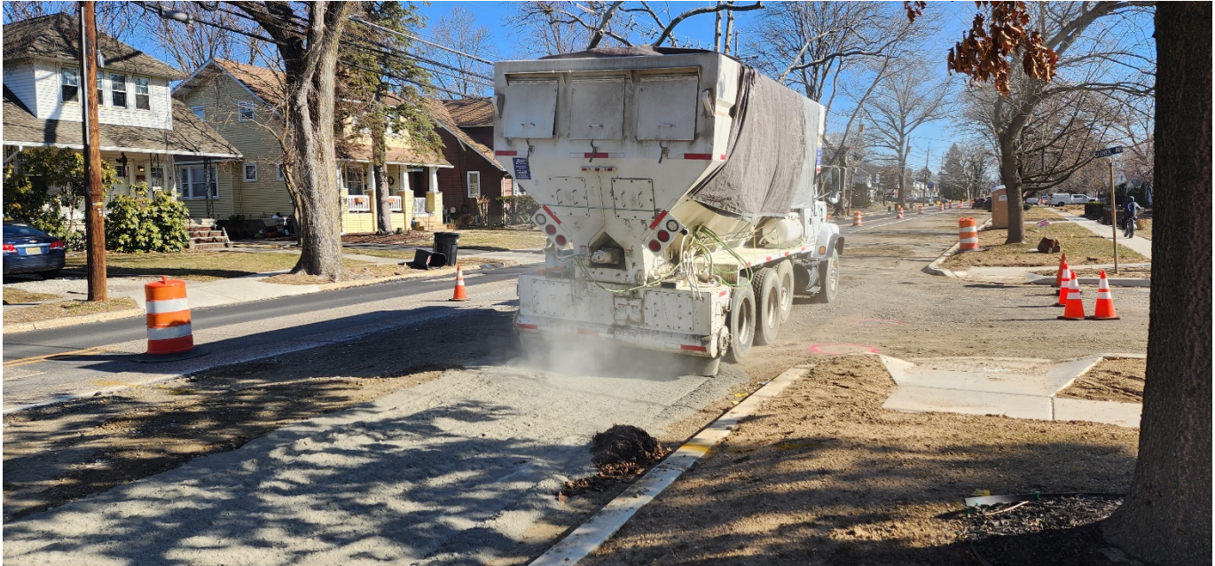
Figure 4: Full depth reclamation in progress
