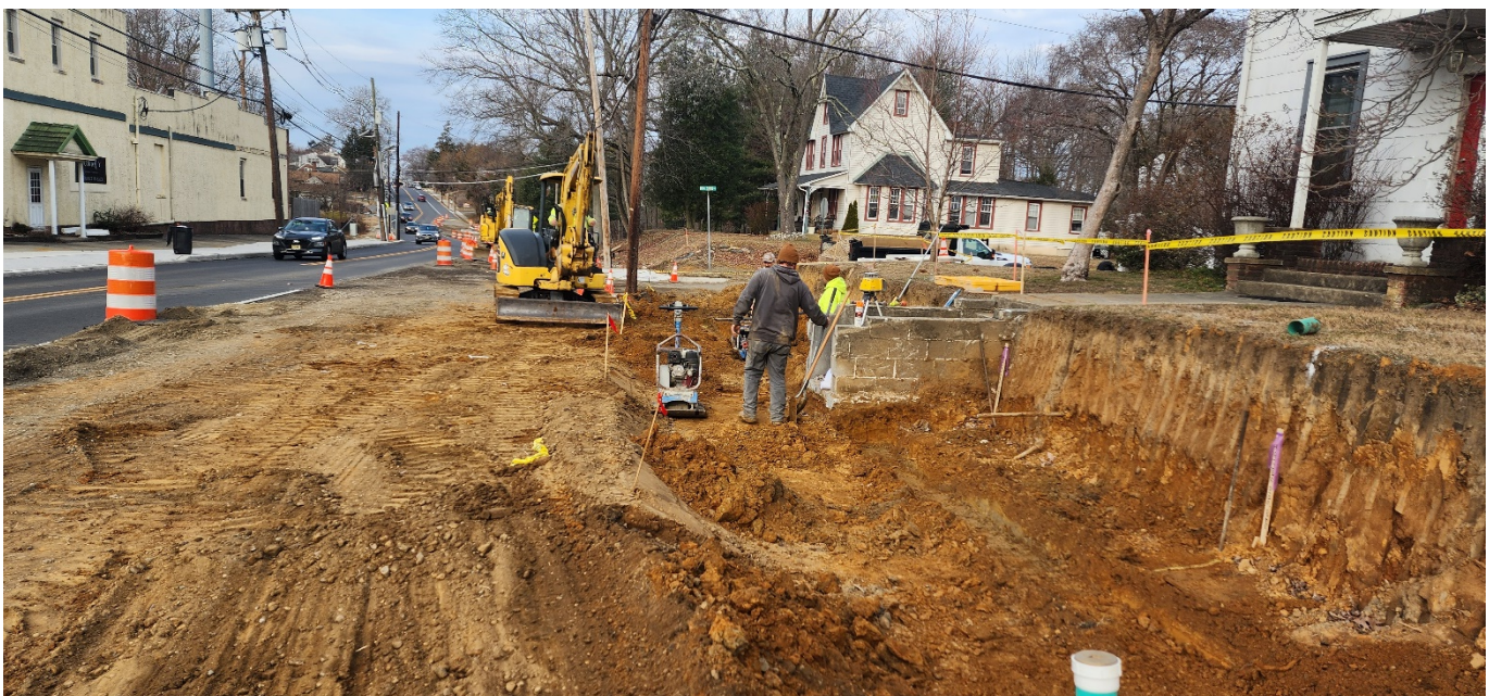
Figure 5: Excavation for retaining wall installation at the corner of Hampshire
